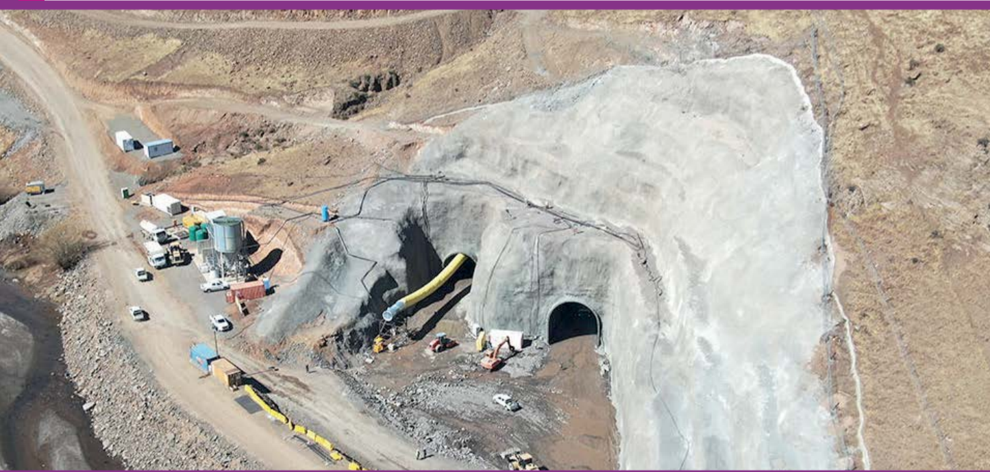
The Polihali Dam in Mokhotlong
