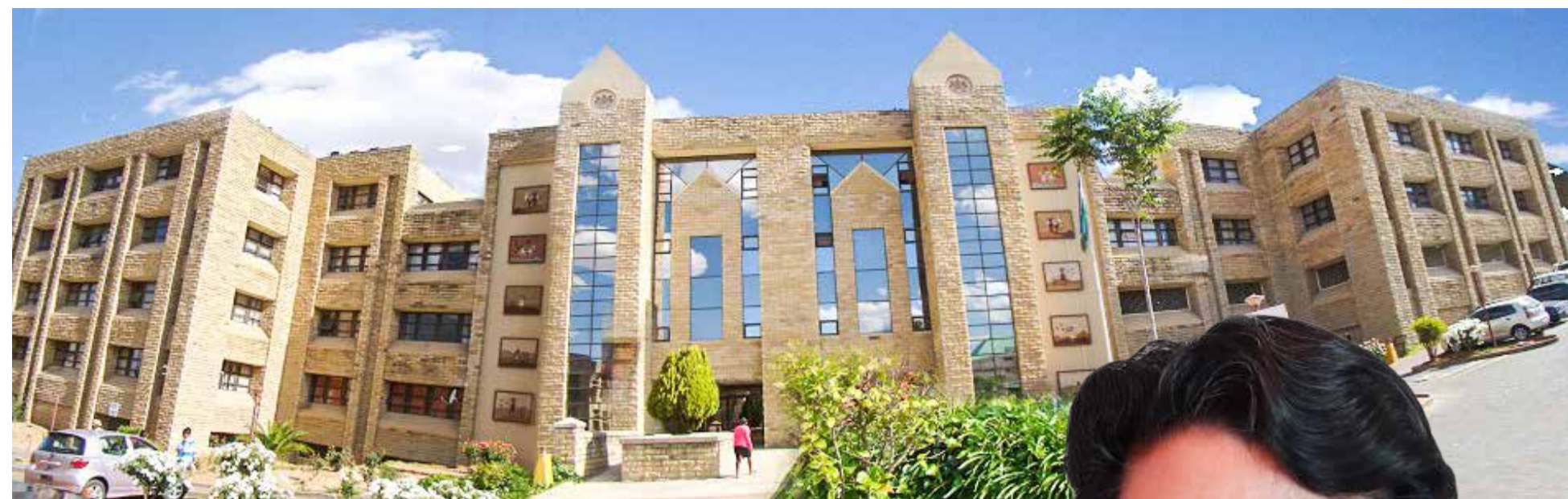
Government office complex, Finance house
